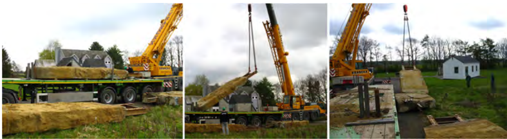
Fig. 5. Arrival of the soil mix panels at the laboratory facilities of BBRI
