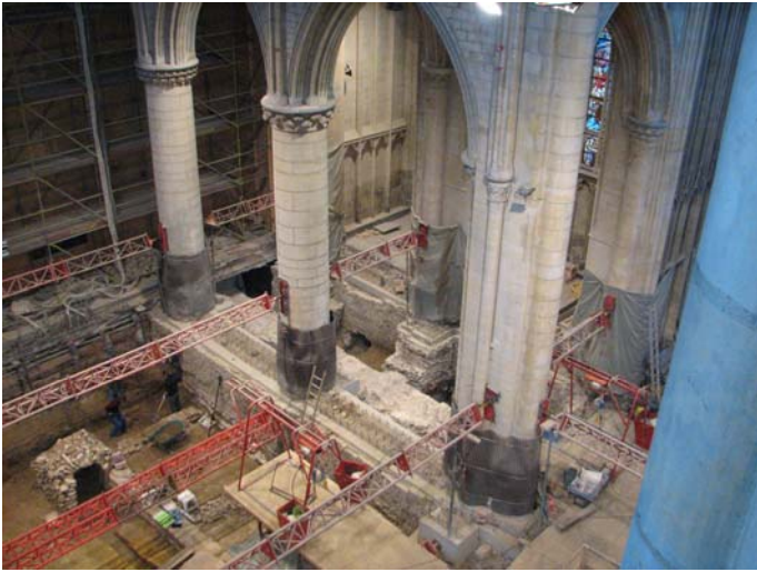
Figure 8: General view of the excavations
